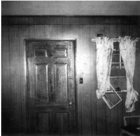
FIGURE 6.3.7.11.2.2 Blistering of Varnish on Door and Slight Scorching of Draperies, the Only Indications of the Natural Gas Flash Fire.
