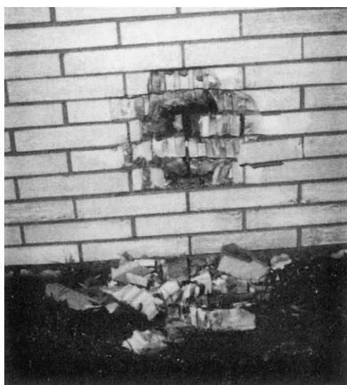
FIGURE 6.2.9.2 Damage to an Outside Brick Wall Caused by Thermal Expansion of an I-Beam in the Basement.
