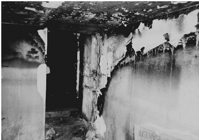
FIGURE 6.3.7.5(b) Truncated Cone Pattern Displayed on Perpendicular Walls.
