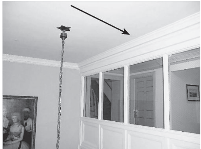
FIGURE F.3(a) Sprinklers to Maintain Glass Cooling.
