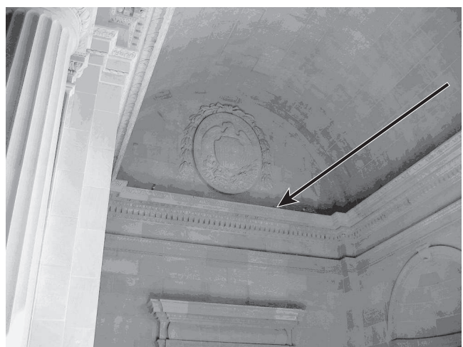
FIGURE F.3(c) Exposed Sprinkler Pipe.
