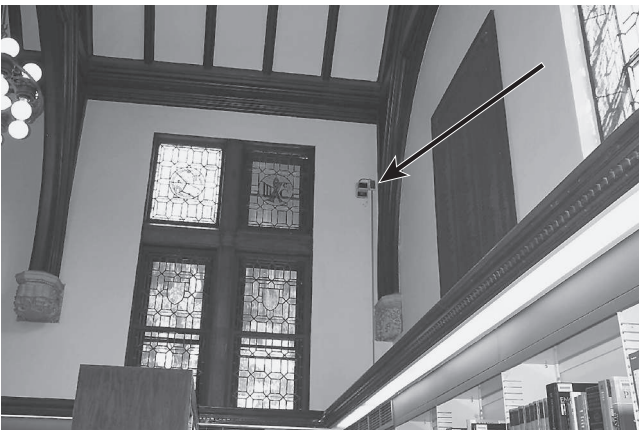
FIGURE F.4(c) Linear Beam Smoke Detector.
