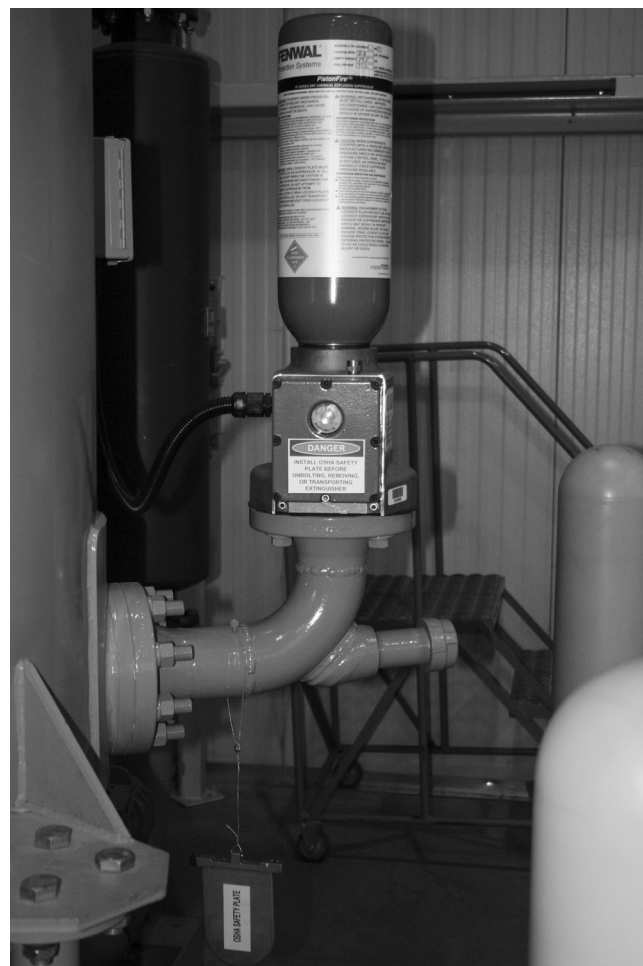
FIGURE 6.2.3.6.3(a) HRD Suppressor with 20 mm HRD Valve.
