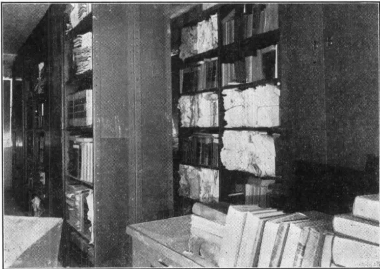
Fig. 5—Record room with 50 lbs. per sq. ft. combustibles. Cement finish floor, metal shelving.
