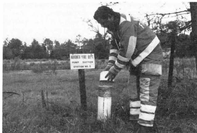
Figure B-5-2.2(a) A dry hydrant innovation has eliminated the top 90° or 45° elbow on each hydrant. (Photo by Nahunta Volunteer Fire Department, North Carolina)
