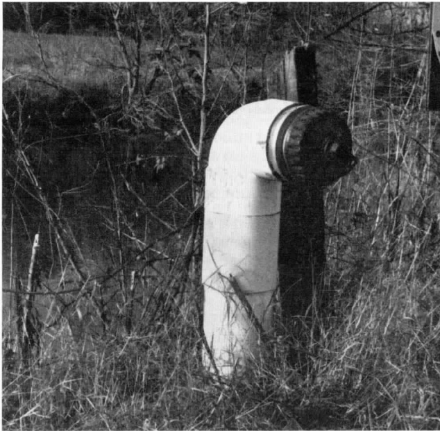
Figure B-5-1(a) Dry hydrant.
