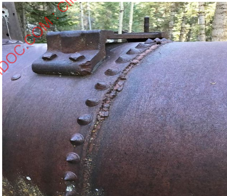
Figure 1-1: Period Repair Work on a Riveted Seam
