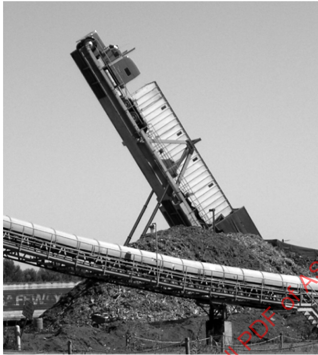
Fig. L-4-1 Interlocked Truck Dumps
